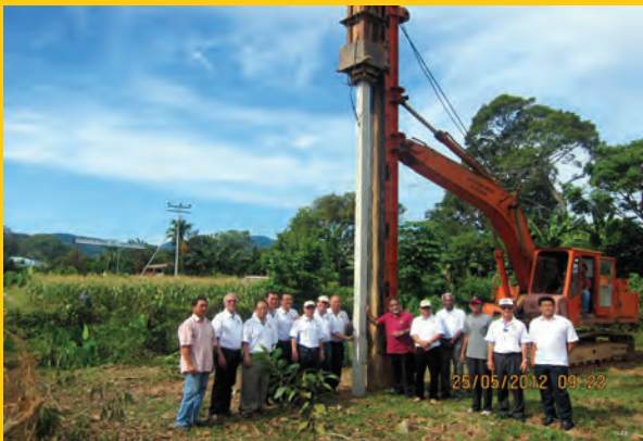
The first pile about to go in.
