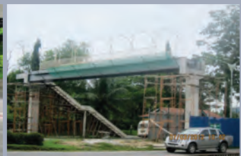
Another project site-overhead pedestrian bridge under construction.
